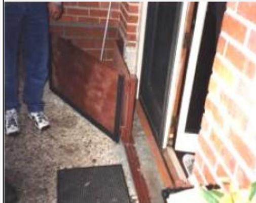
The same house has a removable barrier to block water entering through the opening for the door
